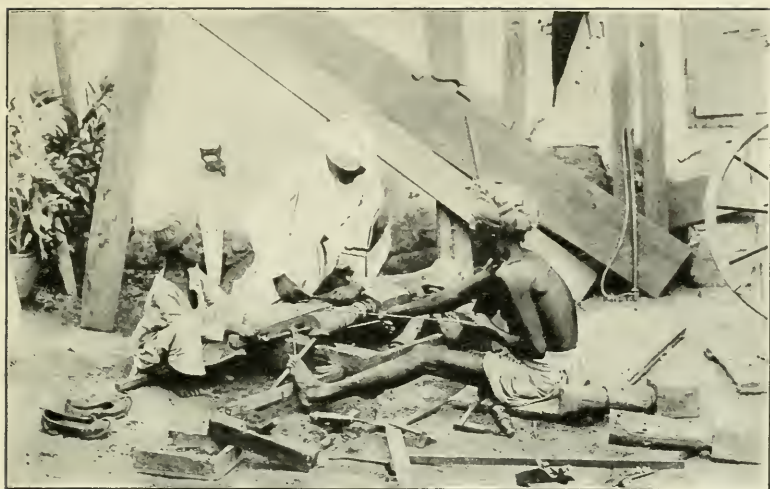
Indian carpenters at work
